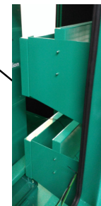
Noise & water proof air intake louvres
